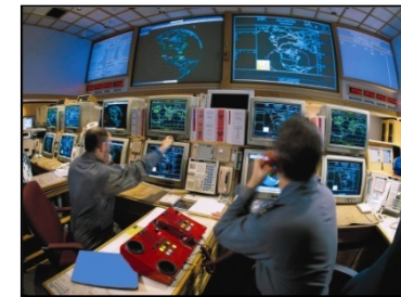
C2BMC Control Room
